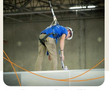
Self-retracting lifelines are connecting devices also known as retractables or yo-yos. Self-retracing lifelines are a valuable and versatile tool for preventing falls. Users must understand how fall arrest systems can prevent deaths and serious injuries. Review the following self-retracting lifeline safety tips with your employees.
