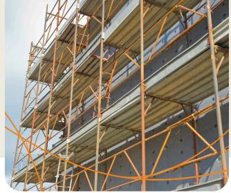
Scaffolds can tip over, collapse or employees can fall through improper planking. Employees on the job site must
